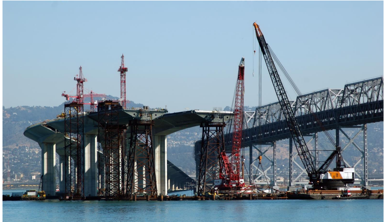
San Francisco-Oakland Bay Bridge
