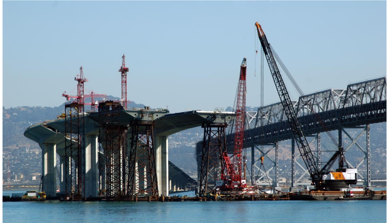
San Francisco-Oakland Bay Bridge
