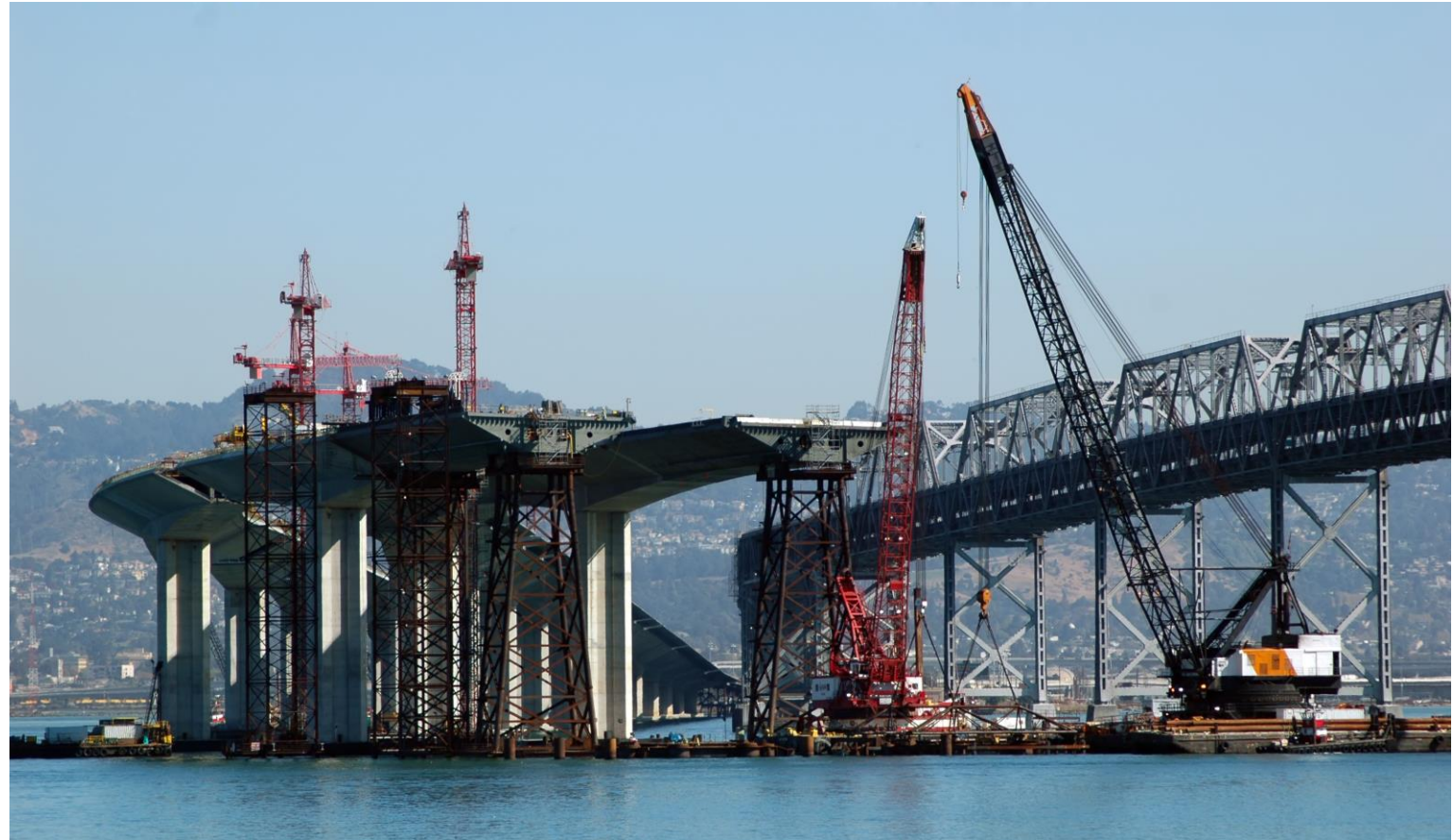
San Francisco-Oakland Bay Bridge
